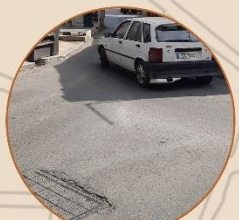
Failure to handle gutters
